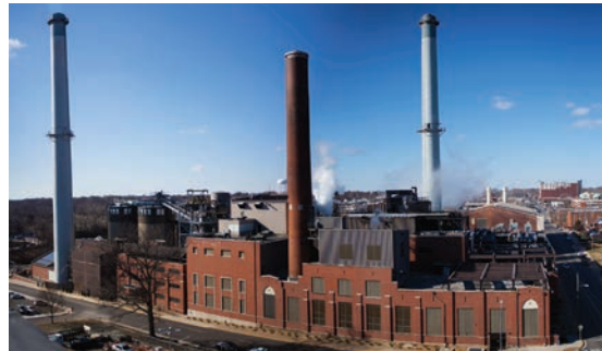
The University of Missouri's combined heat and power (CHP) plant serves heat and electricity to the campus.
